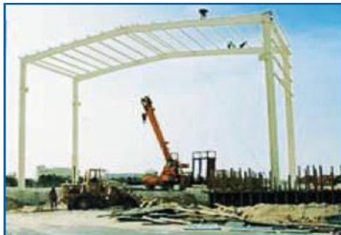
Fixing of purlins
