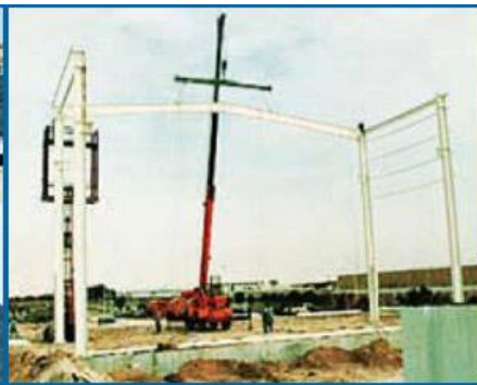
Erection of rafter and columbs
