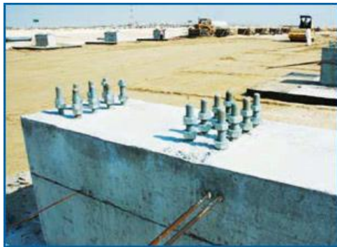
Anchor bolt foundation
