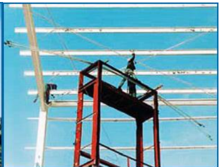
Fixing of roofing bracing
