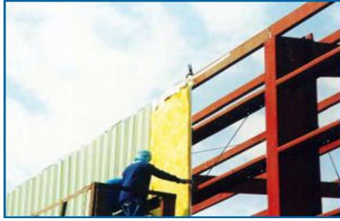
Fixing of insulated wall sheeting
