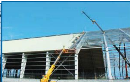
Fixing of roof sheets
