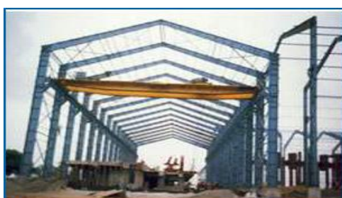
Fixing of crane in shed
